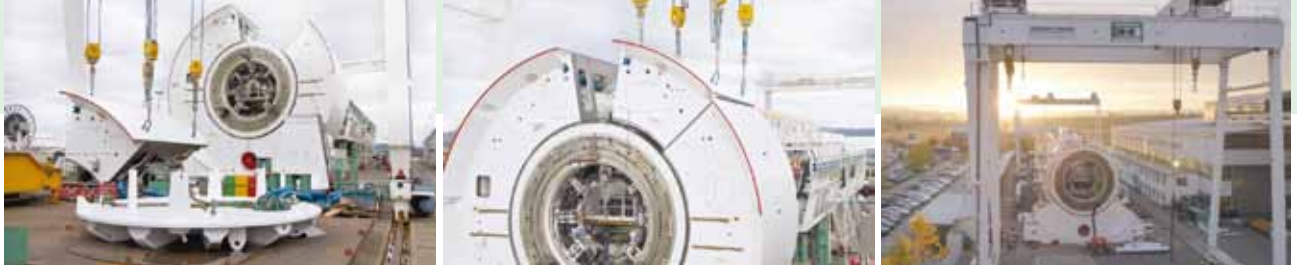
Assembly of the S-574 EPB Shield in Schwanau, Germany .
